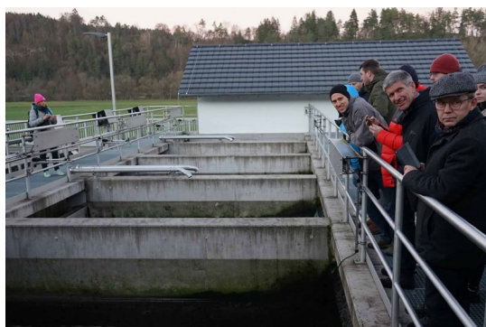
Fig. 7: WWTP Immendingen. Basins for granular activated carbon filtration. © Nikolaos Tzoupanos
